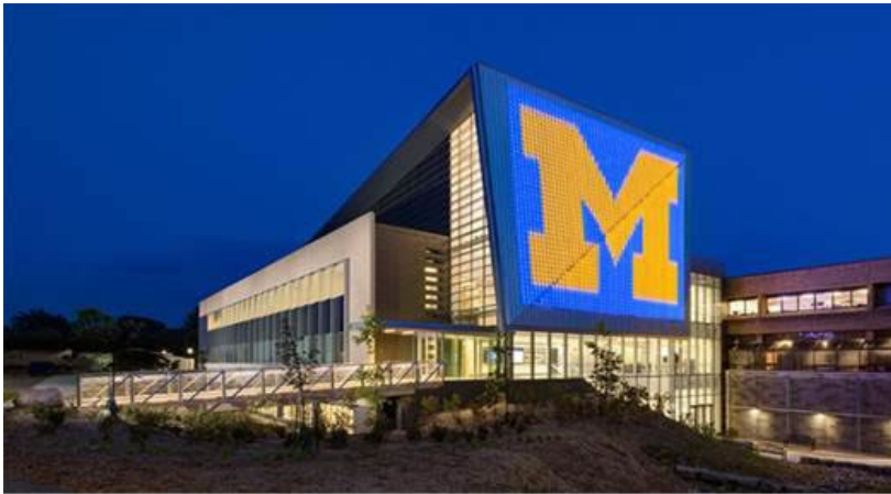
GG Brown Laboratory of Mechanical Engineering addition on the University of Michigan's North Campus in Ann Arbor.
