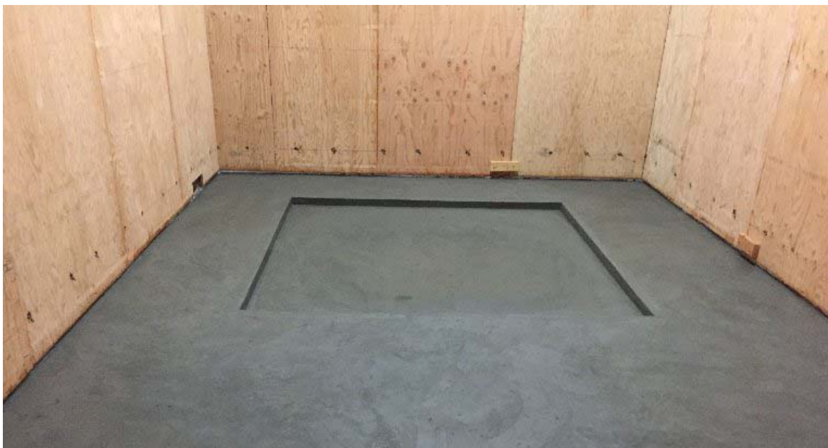
Nion STEM recessed floor. (Image courtesy IMRI)
